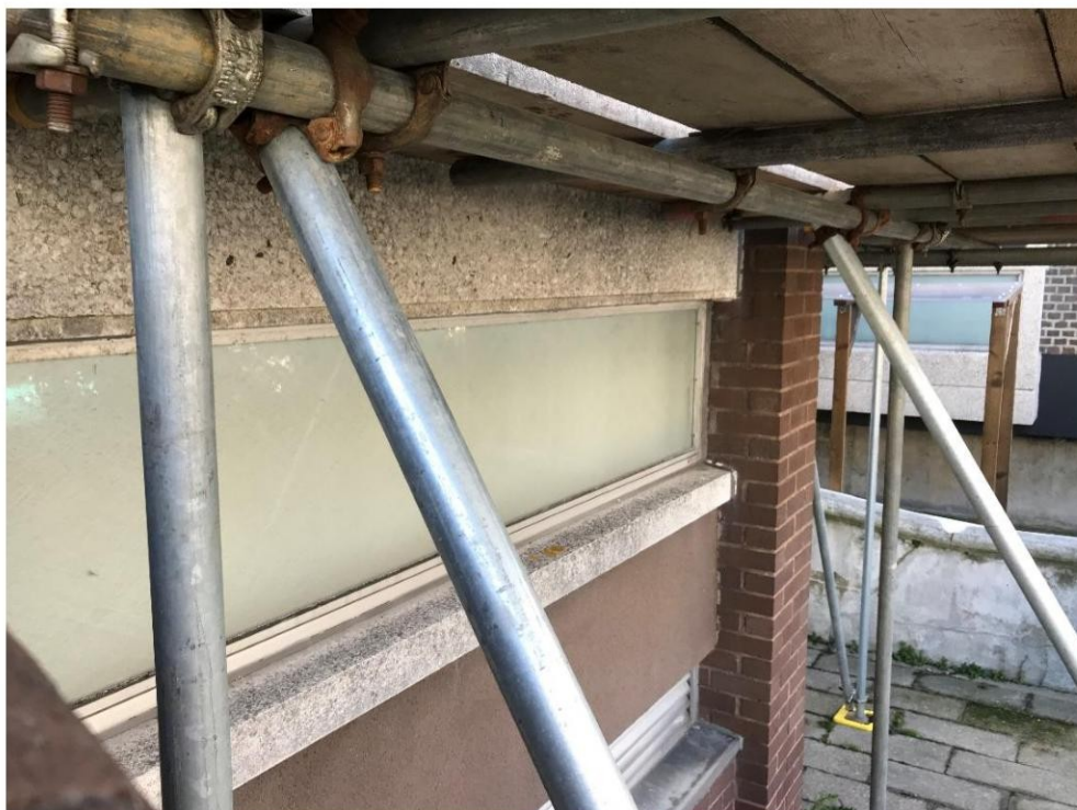
Fig.10 Glazed panels below windows - outside
