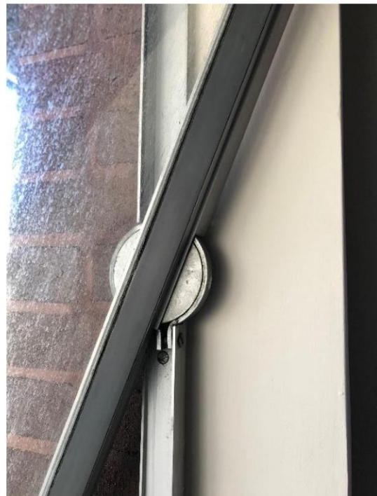
Fig.12 Centre hinge opening window detail - inside
